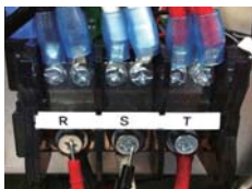
* Measuring input voltage
